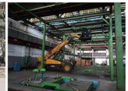
Telescopic Handlers Build Sugar Refinery in Ethiopia
