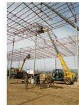
Telescopic Handlers Build Steel Structures Overseas
